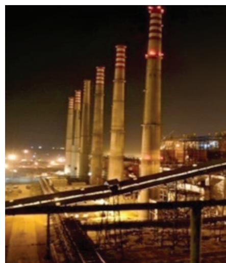
360 KTPA Aluminium Smelter Plant with 900 MW captive power of Hindalco Industries at Singrauli, Madhya Pradesh
